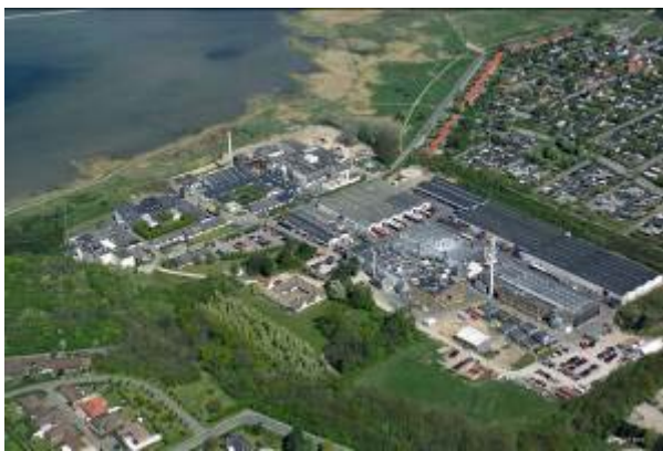
Catalyst plant in Frederikssund, DK
